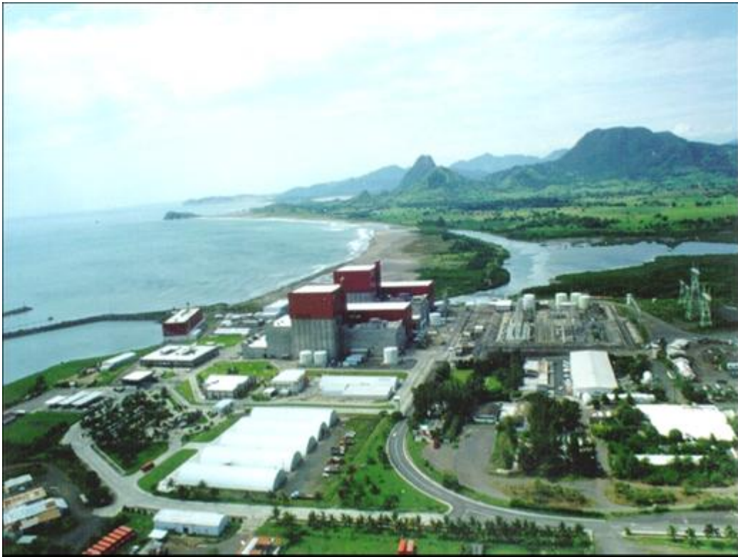
Fig. 3. Laguna Verde Nuclear Power Plant
